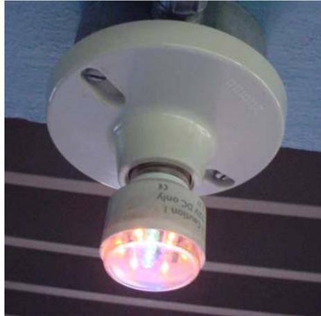
**Figure 6. Steca 0.7 W LED light used in the Honduras PV telecenters.**
