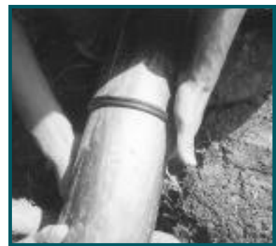
Fusion joining of pipe
