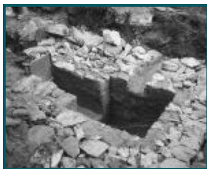
Intake/Forebay under construction
