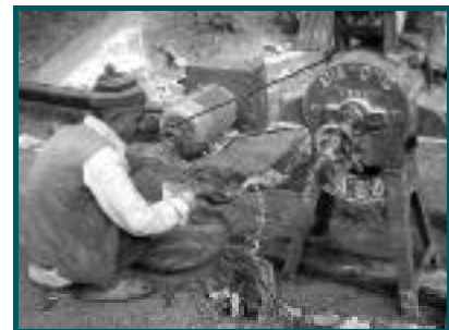
Installation of Mill
