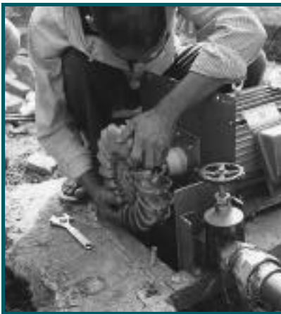
Attachment of turbine to generator shaft
