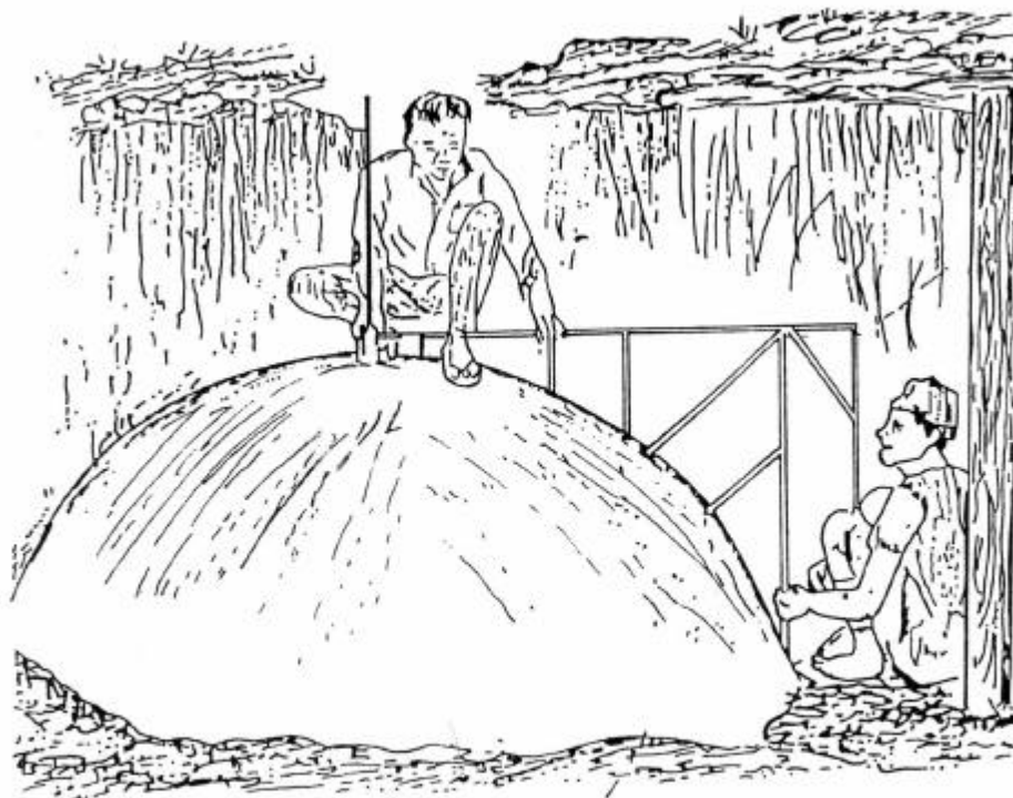
FIGURE - 9-4 MAINTAINING REQUIRED SHAPE OF THE DOME WITH THE HELP OF A TEMPLATE
